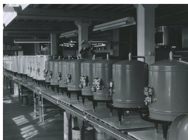
Hatco booster assembly line
