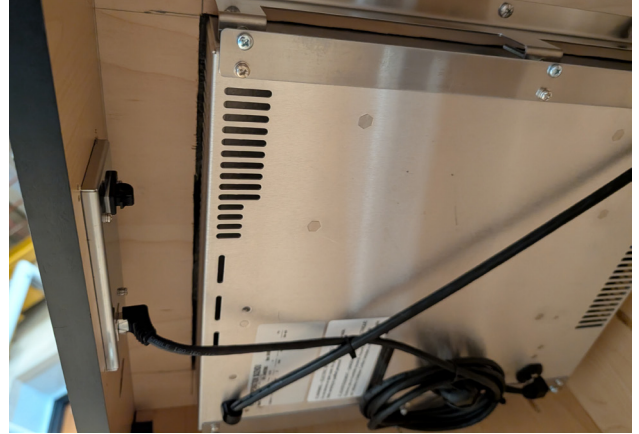
Typical installation with substrate under countertop.
