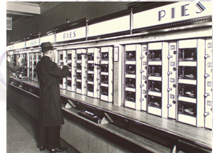
Photo courtesy of the New York Public Library
